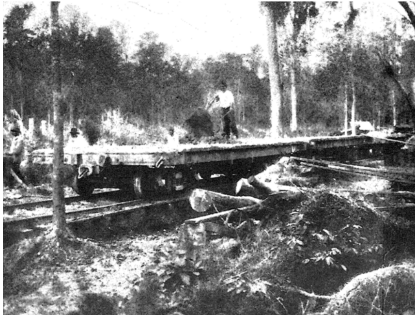
Figure 22. Loading phosphate rock for transport to the washers. Top photograph shows loading into a hopper with the tram adjacent to pits ( http://www.angelfire.com/sc2/tokenofthemonth002 ). Bottom photograph shows loading from wheelbarrows onto a flat car (Waggaman 1913).
