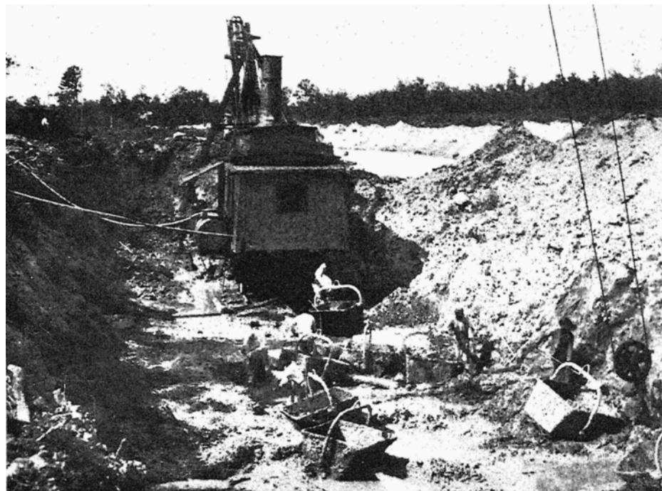
Figure 23. Land mining with steam shovels. The top photograph shows the shovel removing overburden and depositing it on either side of the pit. The lower photograph shows the subsequent phase of removing the phosphate rock and loading it in buckets that were then lifted out of the pit and dumped in rail cars (Waggaman 1913).
